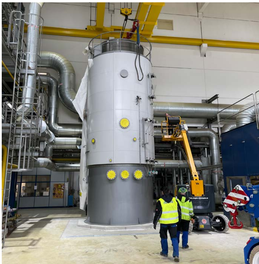
Electric boiler for steam production being installed
