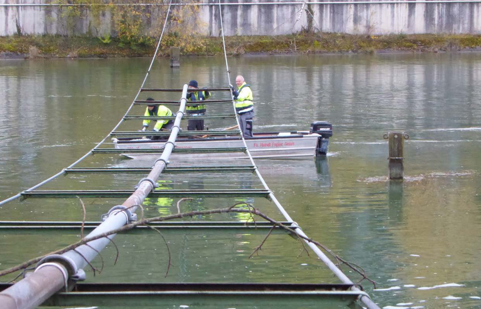
Dismantling of the irrigation pipes in the water basin to protect waterfowl.
