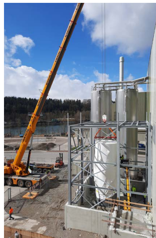
Installation of an electric boiler for steam production.
